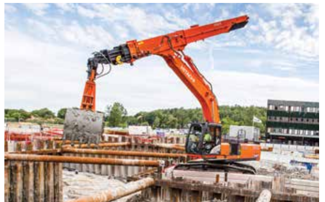
Special application excavators
