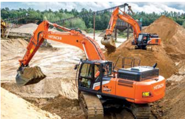
Zaxis medium excavators
